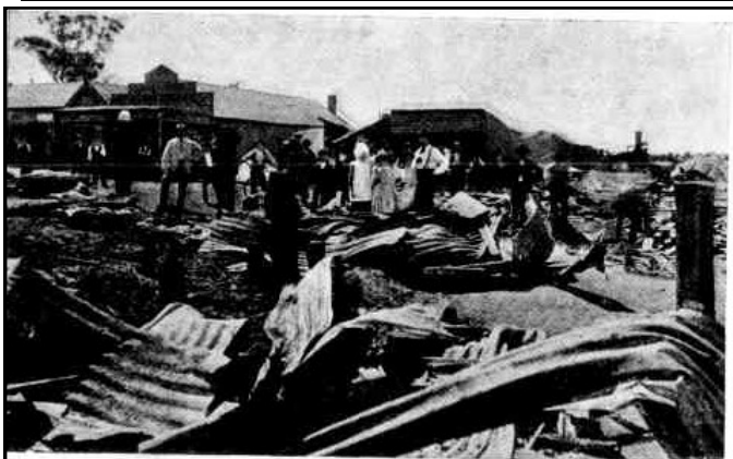
LOOKING FROM REAR OF BASHA'S, SHOWING FRASER'S, MCGILL'S, CRAIG'S, AND O'KEEFE'S.
